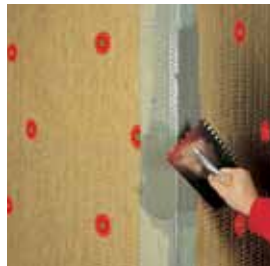
— Reinforcing a corner
