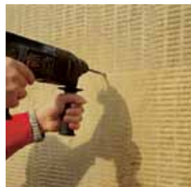
— Drilling a hole with a drill
