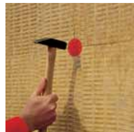
— Hammering the anchor in its place
