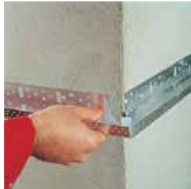
— Measuring profile height and placing it
