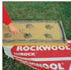
— Applying Kale Mantotech Thermal Insulation Board Adhesive Mortar on points.
