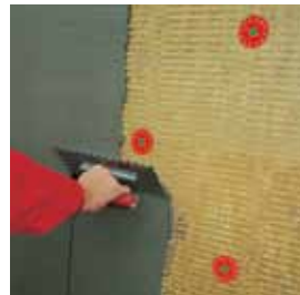
— Smoothing adhesive mortar with the smooth side of the trowel
