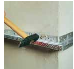
— Installing profile and fixing with screws
