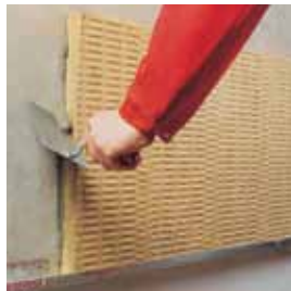
— Removing surplus adhesive
