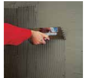
— Applying the adhesive mortar with the notched side of the trowel
