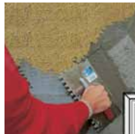
— Preventing danger of cracking
