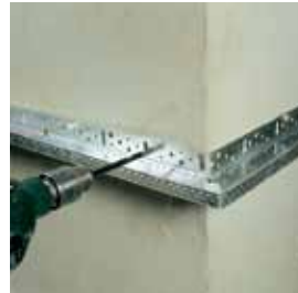
— Drilling holes for screws
