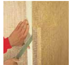
— Cutting off surplus insulation in the corner
