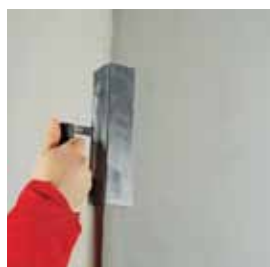
— Reinforcing and smoothing the corners
