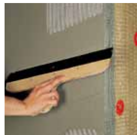
— Applying Kale Rockwool Reinforcement Mesh
